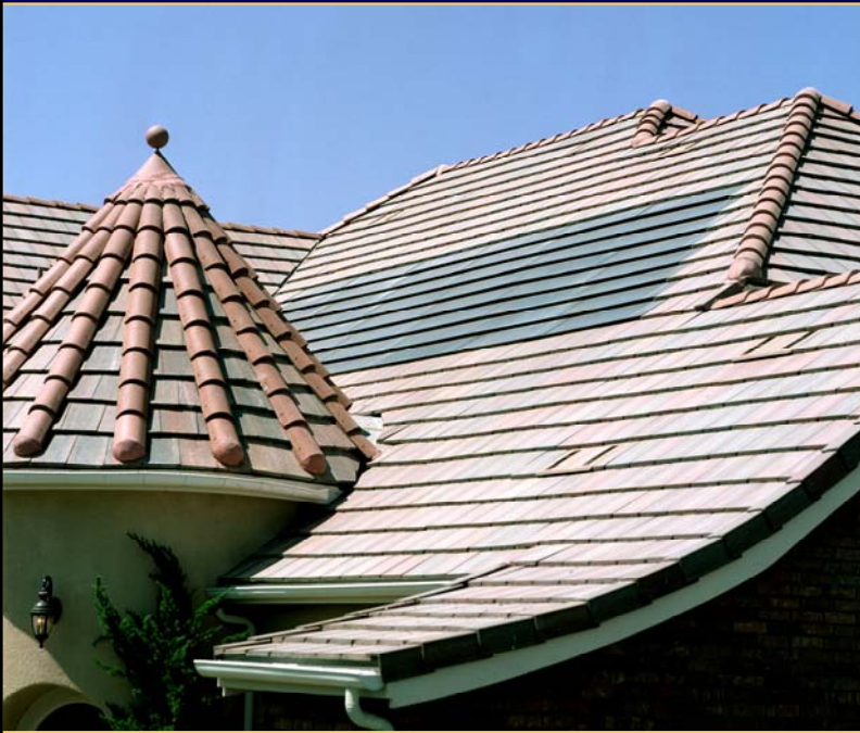
With concrete roof tiles
