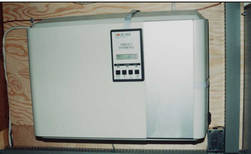
2 kW ARISE GX 5000 inverter.
