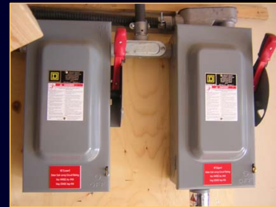
DC array switches
