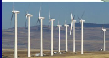
Electricity generating plant
