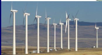
Electricity generating plant
