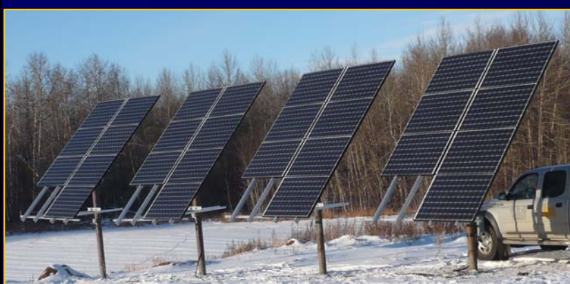
5 kW solar PV system Dave Shiflett house near Devon Connected to Fortis Alberta
