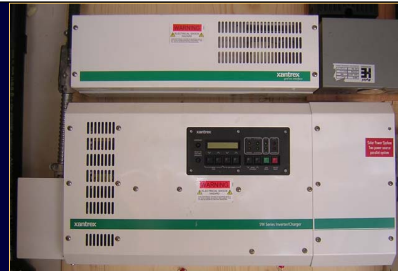
Xantrex Inverter /charger
