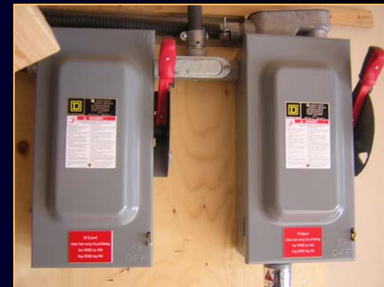
DC array switches
