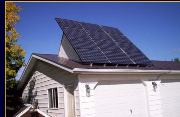
2.4 kW solar PV system Mel Krisher house near Sangudo Connected to Central Alberta REA
