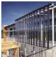
An active solar hot water system serves as a source of heat for the building.
